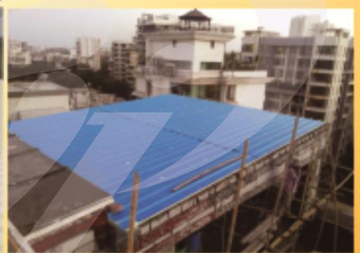
Residential site at Juhu on 7th floor
